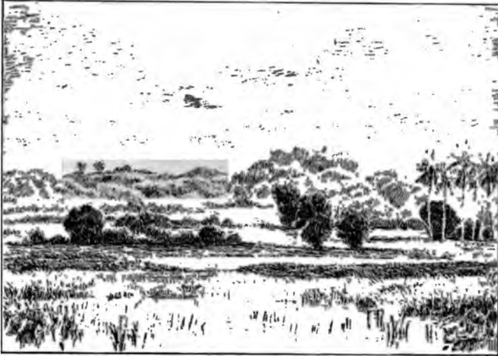
SEWAGE FARM ON THE BEACH, LOOKING INLAND FROM THE MARINA.
